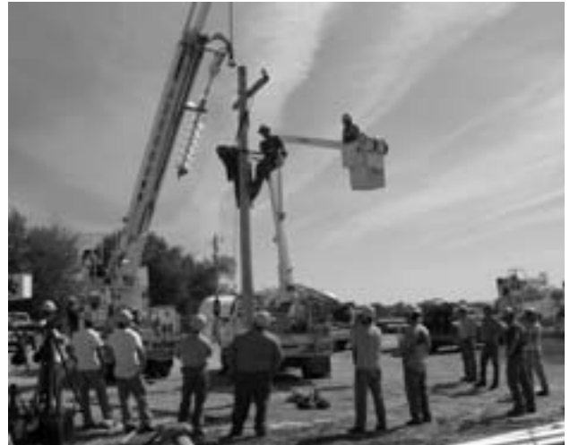
The Brooklyn and Sigourney linemen are shown above reviewing the procedures for pole-top rescue.
