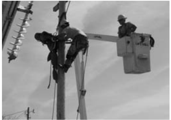
Jordan Terwilliger, an Apprentice Lineman on our Brooklyn crew, practices his pole-top rescue.
