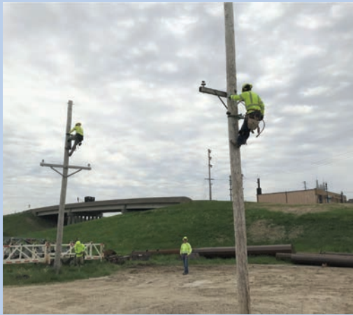
Pictured above are linemen practicing their pole climbing competency.
