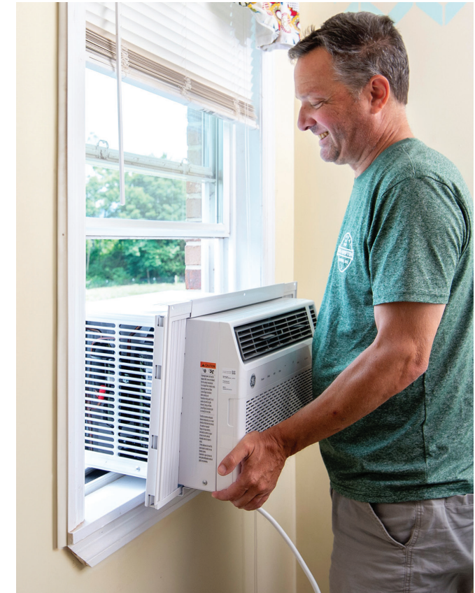
Removing any window AC unit for the winter months prevents heat from escaping your home and wasting energy. Add this to your annual fall winterizing chore list to help save money.
